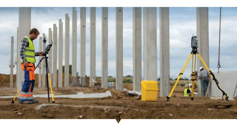
Trimble VISION technology integrates calibrated digital cameras with Trimble S9 and S7 total stations, as well as the Trimble SX10 scanning total station. These instruments have the ability to collect survey data, stream video from the perspective of the instrument, and capture panoramic still images. Trimble Access field software overlays survey data on the streaming video, which enhances your field productivity when operating the instrument robotically.
